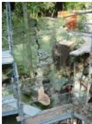
The phases of intervention of restoration the Uccelliera, with the demolition of the large oaks near the arches and the consolidation of the same with belts of carbon fibers.
