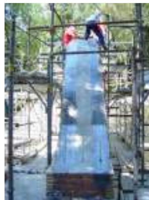
The phases of intervention of restoration the Uccelliera, with the demolition of the large oaks near the arches and the consolidation of the same with belts of carbon fibers.
