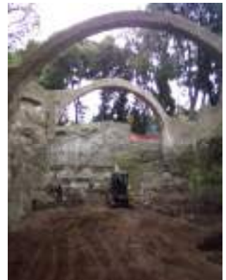
The phases of intervention of restoration the Uccelliera, with the demolition of the large oaks near the arches and the consolidation of the same with belts of carbon fibers.
